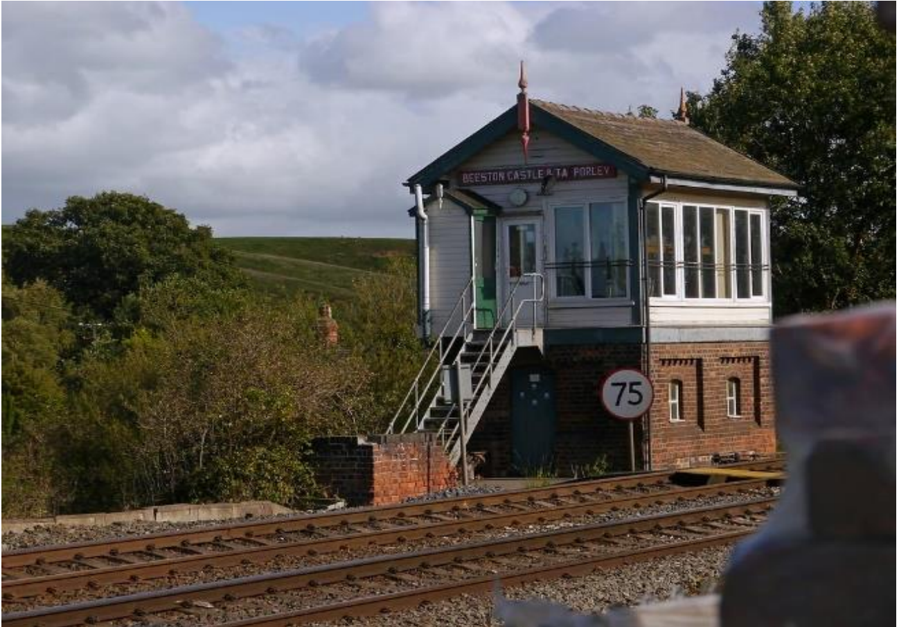
Figure 2 - Existing signal box at the site
